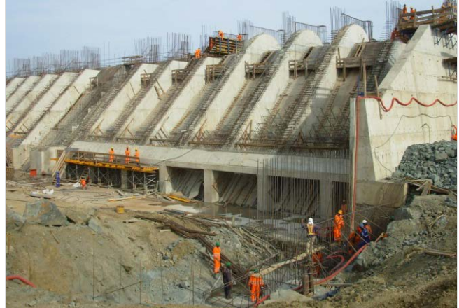
View of the Bujagali power plant under construction
