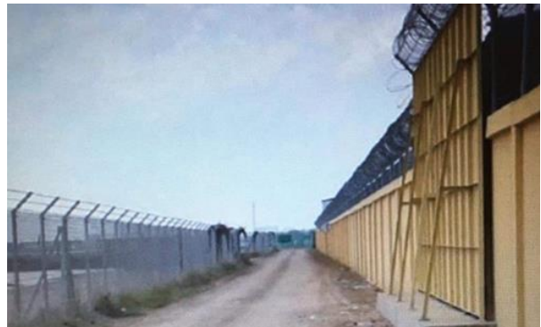
New airport interior fence and refurbished exterior boundary wall.
