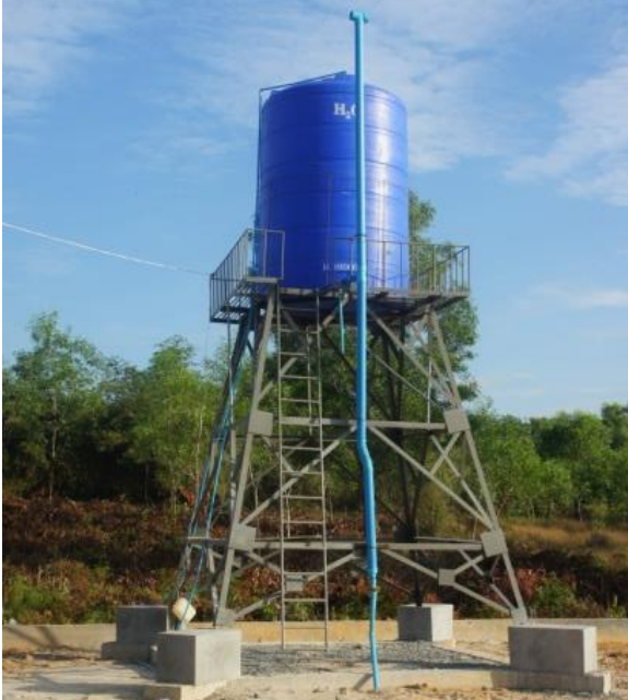
Water system at the new relocation site – “Meanchey Development Community”
