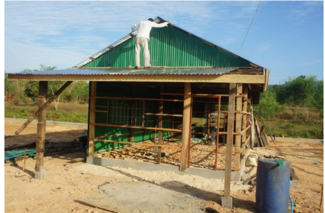
New home under construction at Meanchey Development Community
